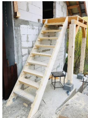
Stairs to the new room
